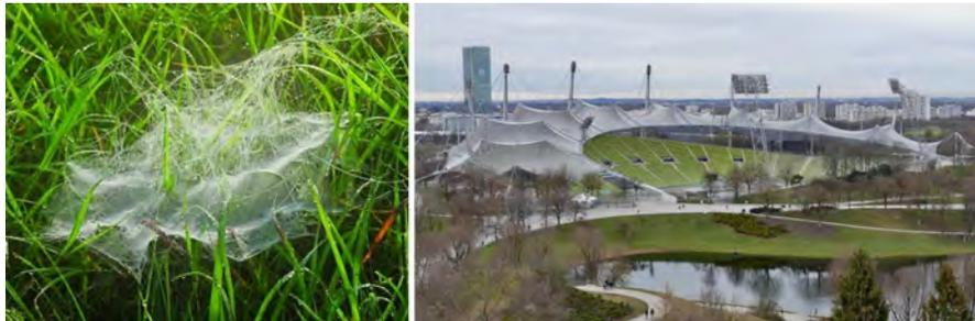
**Fig8.** Example of analogy: The roof of the Munich Olympic Stadium was inspired by natural structures such as cobwebs
